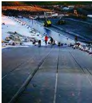
Appearance of geomembrane (asphalt sheet)
